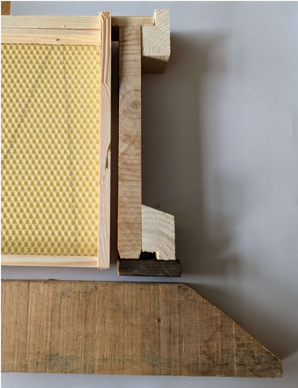
Cross section of a brood box. Entrance here is made with the dark wood, showing the elongated entrance tunnel.
