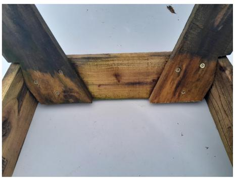
The legs are screwed and glued in place. Notice how the notch in the leg is resting on the crosspiece of wood. This helps to take some of the pressure off the three screws a bit.
